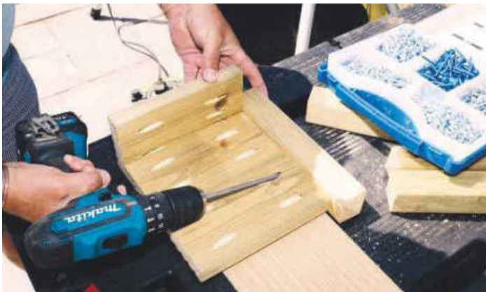
STEP 11. Using an MDF packer, the boards are screwed in – note the decking spacer for the board position
